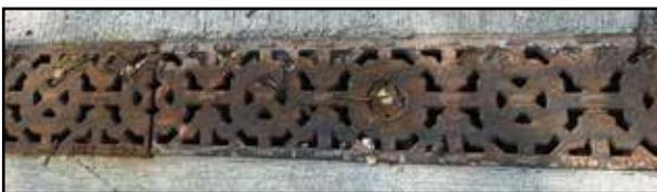
Narrow, deep, filter strips with grass, gravel, or grillwork can be installed along regular paving to interrupt flow.
